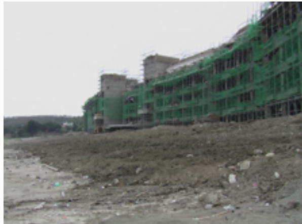
挖方堆置沙灘9
